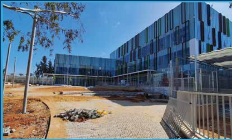
Evan & Layla Green Family Foundation Gogya Building
